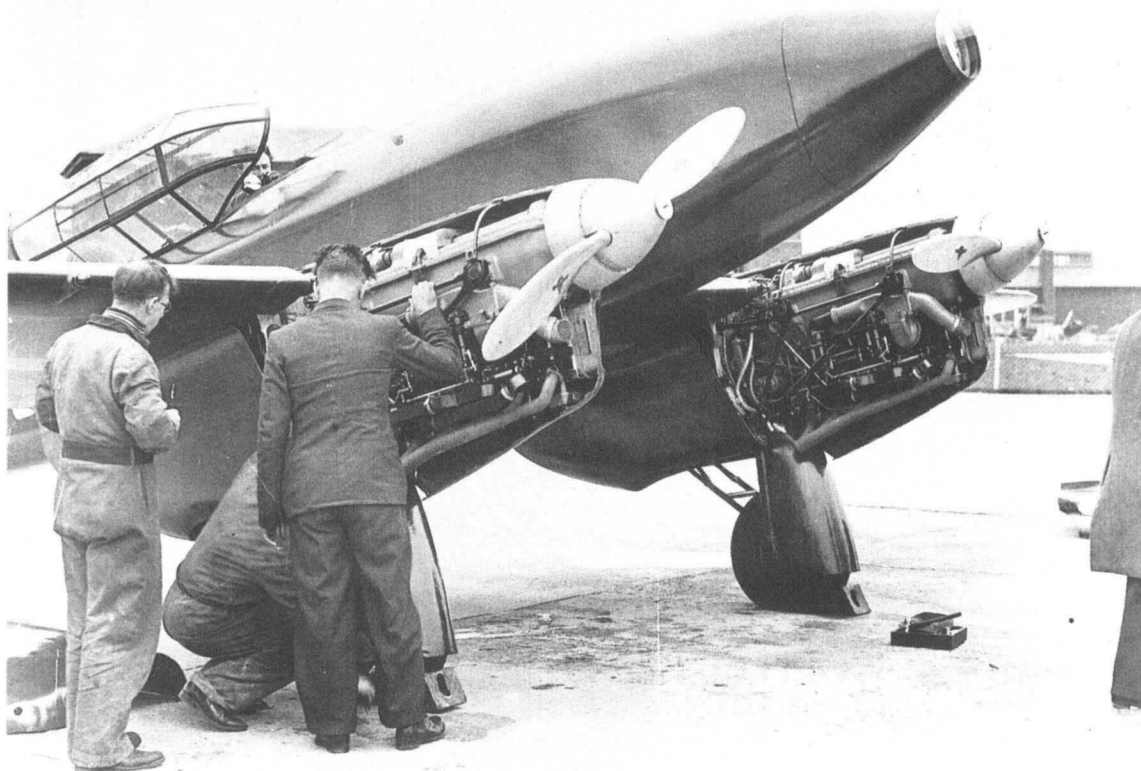
Left: Biggest de Havilland piston engine, the Gipsy Twelve (RAF Gipsy King) was made only in small numbers (about 95). Halford was distressed that it weighed over 1,000 lb.
